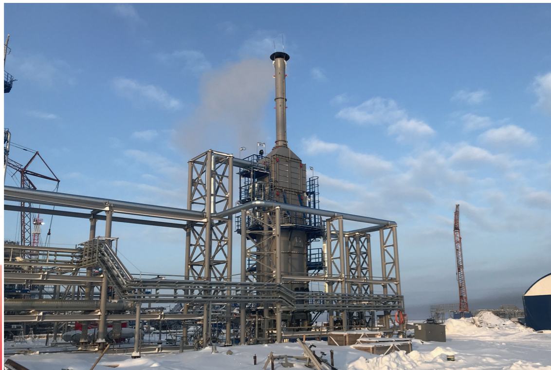
CA-1-106-6-7 Vertical Circular Heater
