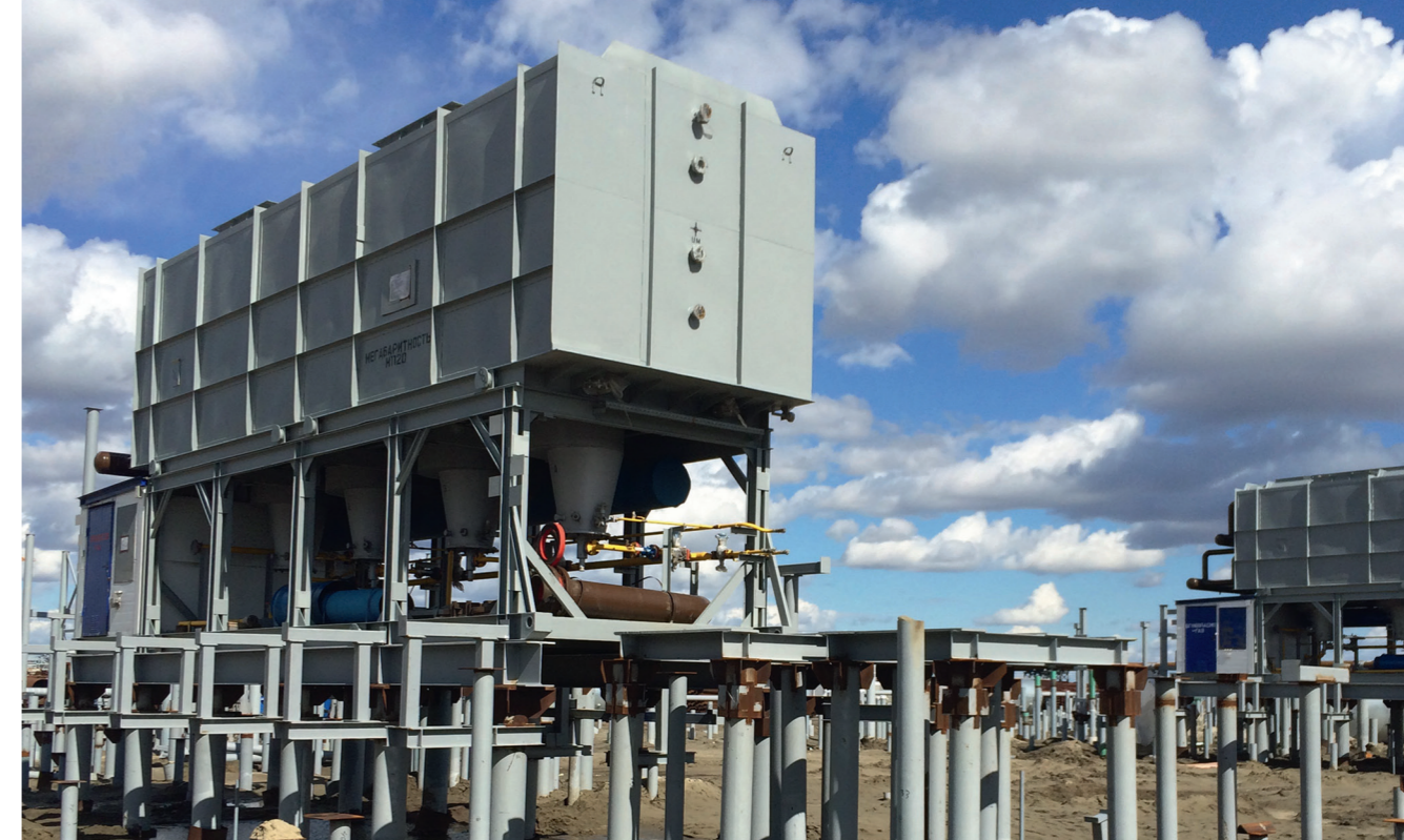
Installation of PTB-5 Tubular Block Furnace at the client's facility
